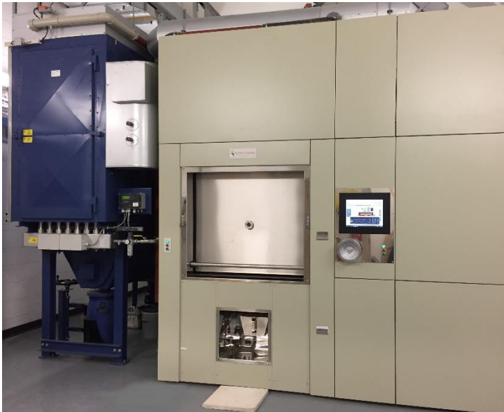
Figure 1 - Typical arrangement showing Bag Filter
